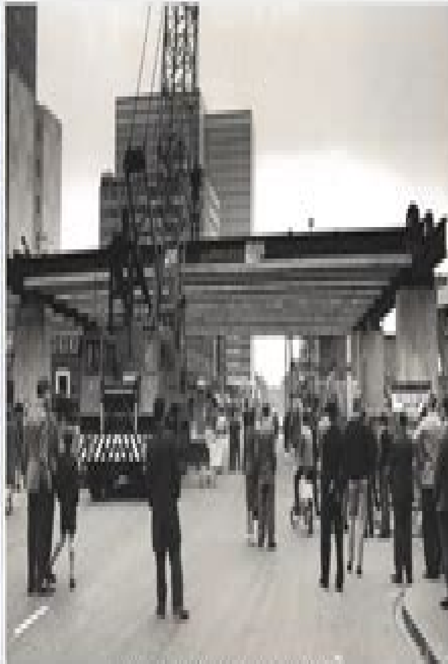
Profess Deans over High Street - Flyover 1967
